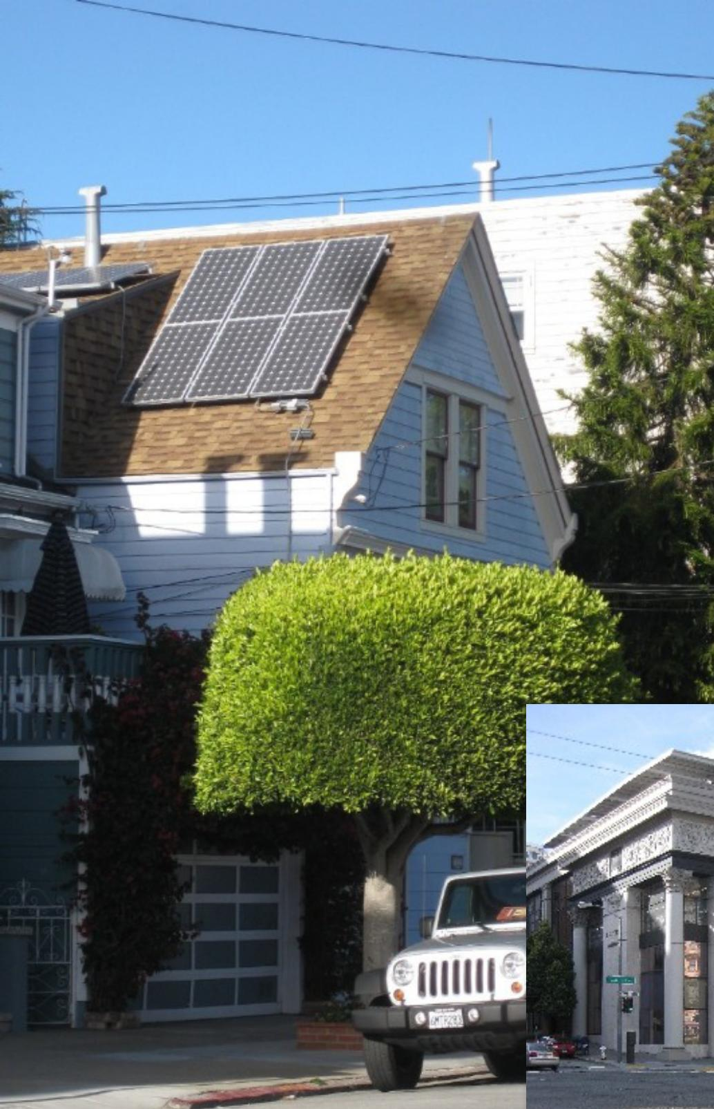
This installation is typical for a modest urban home. Including cells on the remainder of the roof this would be sufficient to power the home. In most cases the installation can be done in a few weeks.
