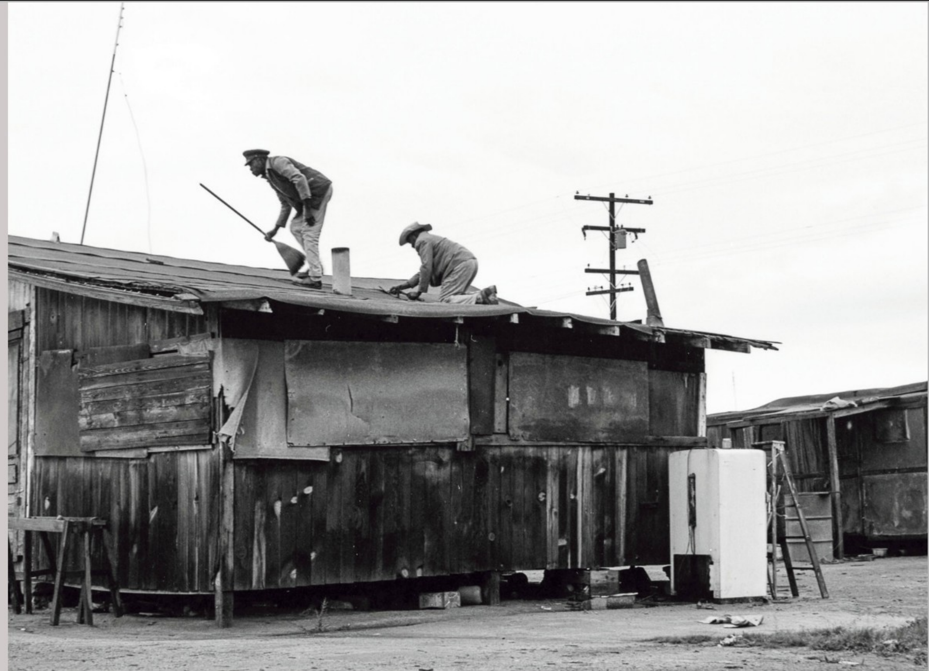
After the storm a homeowner and friend repaired his roof. November 19, 1961
